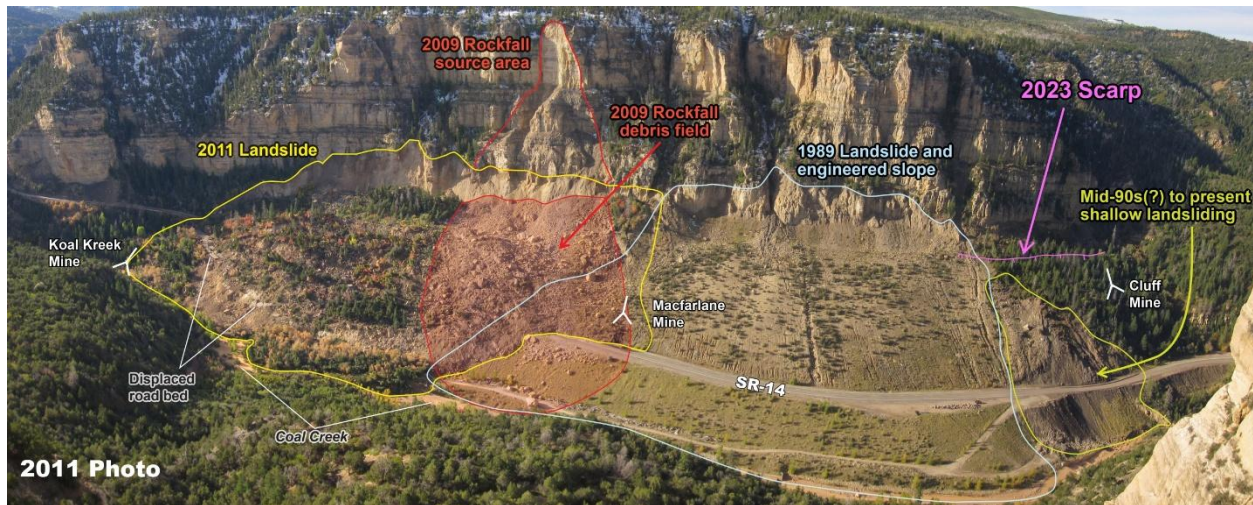
Figure 31: Cedar Canyon, MP8 Landslide Complex, Iron County 77
