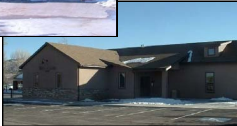
Hatch Community Center
