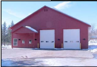
Alton Town Fire Station
