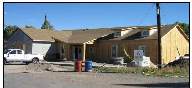
Town of Hatch Multi-Purpose Community Center Under Construction
