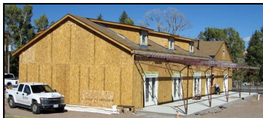
The Town's American Bicentennial picnic pavilion has been re-purposed as a porch covering for the new community center.
