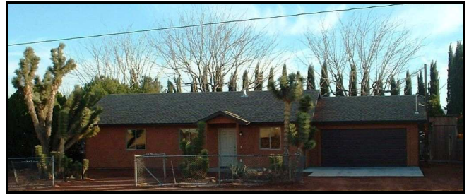
Jane's New Replacement Home
