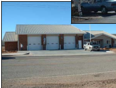
Hurricane City Fire Station Brentwood Area
