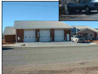
Hurricane City Fire Station Brentwood Area
