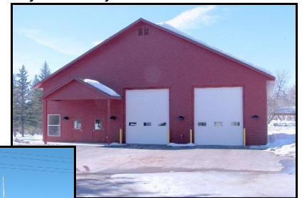
Alton Town Fire Station
