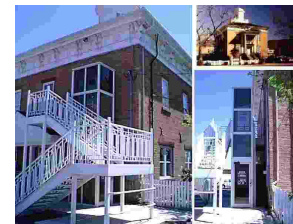
Wheelchair List (ADA accessibility) Pioneer Courthouse, St. George City
