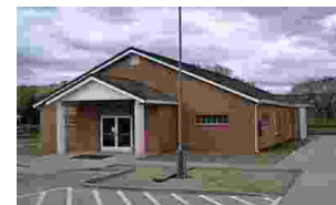
Cannonville Community Center
