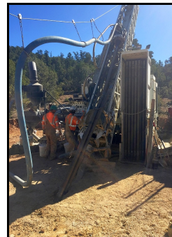
Close-up of the drilling rig.
